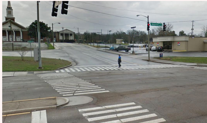
East Magnolia at Kirkwood Street is part of a roadway corridor on the City of Knoxville's HIN.
